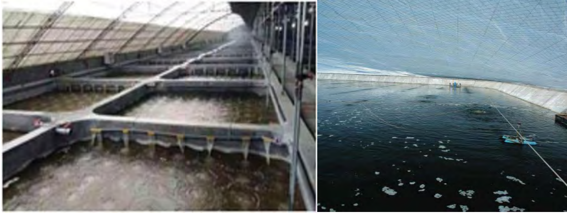
Fig. 8. Green houses for shrimp farming in northern People's Republic of China – a growing operation concept. The facility can provide a well-controlled, natural biosecurity barrier.
