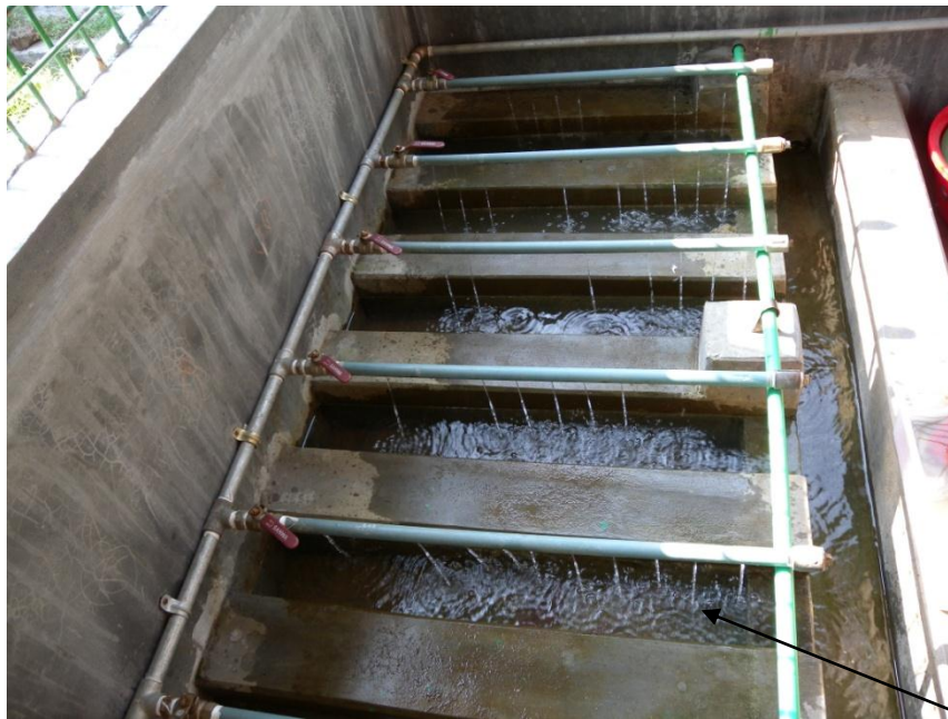
Fig. 1. Small raceway with horizontal perforated pipes to provide continuous flow of sprayed water.
